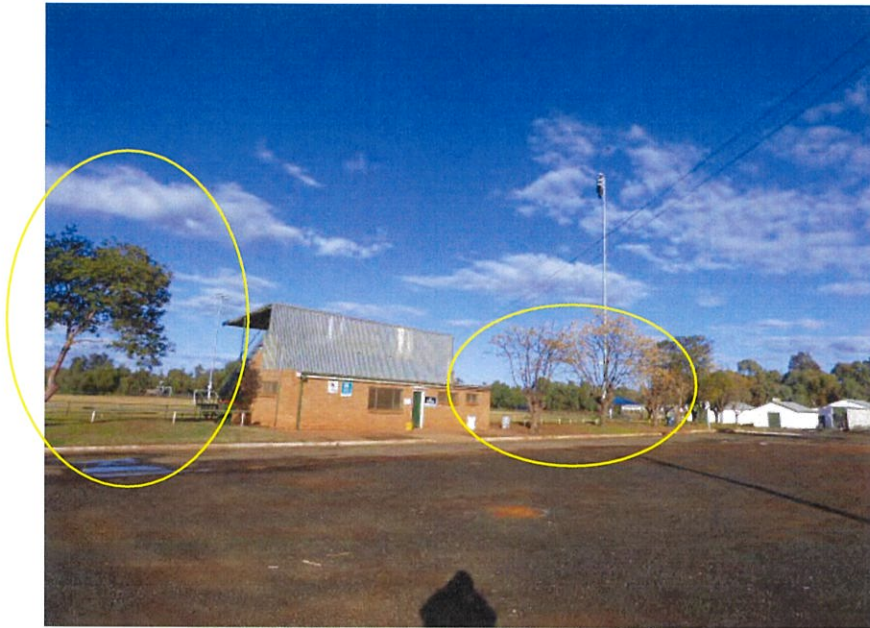
Photo 2 – Area of Car park that forms the north area of the development site, with existing pavilion in middle of shot and the other buildings to right that are to be refurbished. Proposed building encroaches heavily on circled trees – tree numbers 27 – 31 – right side circle. Tree 32 to left of building and as per photo 3 below.
